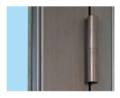
**DISCREET:** thanks to the application to the wood, the straps are completely hidden by the outer aluminium profile and only the central body of the hinge is visible.
